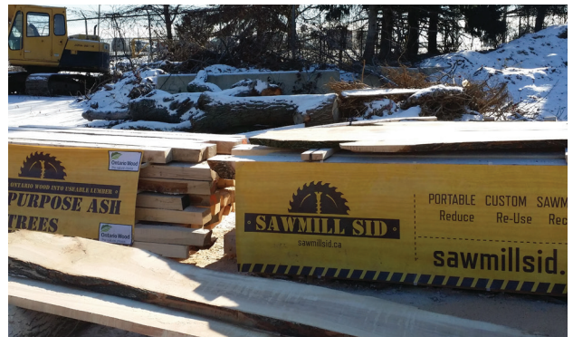
After: Locally Sourced Lumber
